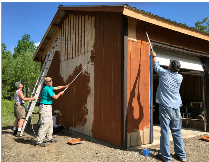
All hands on deck for staining the wood at "Dave's Depot."
