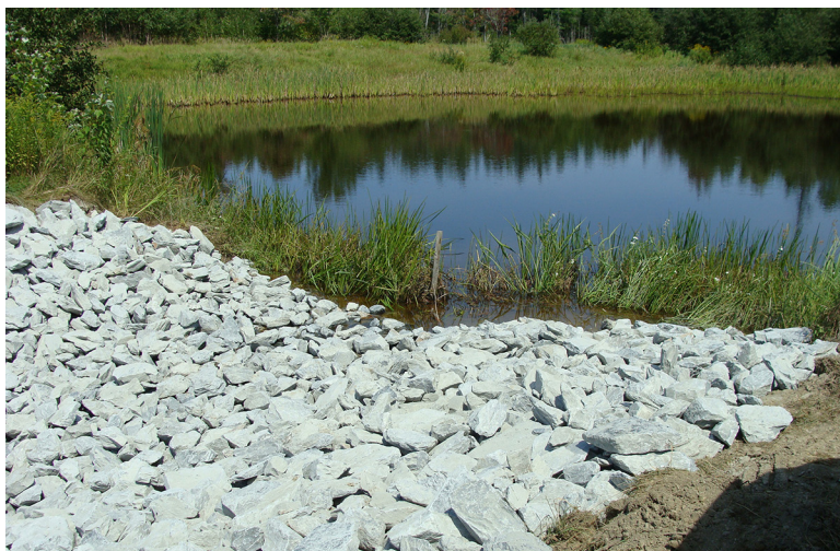
Rip-rap replaced concrete structures. Photo by Sue Owen
