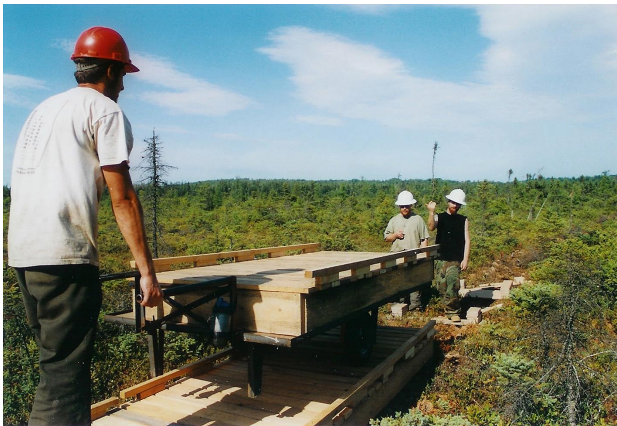
Fig. 19. Arriving with a section at end of incomplete boardwalk. The pair of MCC members in the bog have prepared footings for supporting the arrived section. Ron Lisnet UM photo.
