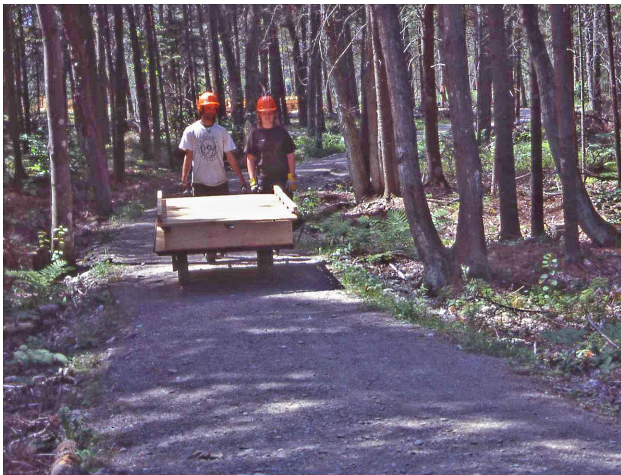
Fig. 13. Transporting a boardwalk section on a special cart along the trail from the assembly site to the incomplete boardwalk. Ronald B. Davis photo.
