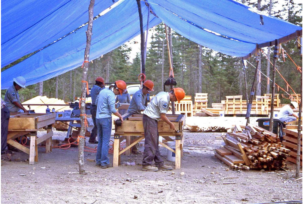
Fig. 15. Maine Conservation Corp crew members at assembly site in summer 2002. Member in central foreground is spiking an end joist on a boardwalk section (see Fig. 6) using a small sledgehammer (zoom in). The incomplete section rests in a jig supported on sawhorses. An incomplete section in another jig is at far left. Its middle joist is in place. The heads of three spikes can be seen on the end joist (zoom in). A pile of bump railings is on the right. Stockpiled components of interpretive stations including railings (see Fig. 8) occupy right background, and a pile of large dimension lumber rests in far-left background. Ronald B. Davis photo.
