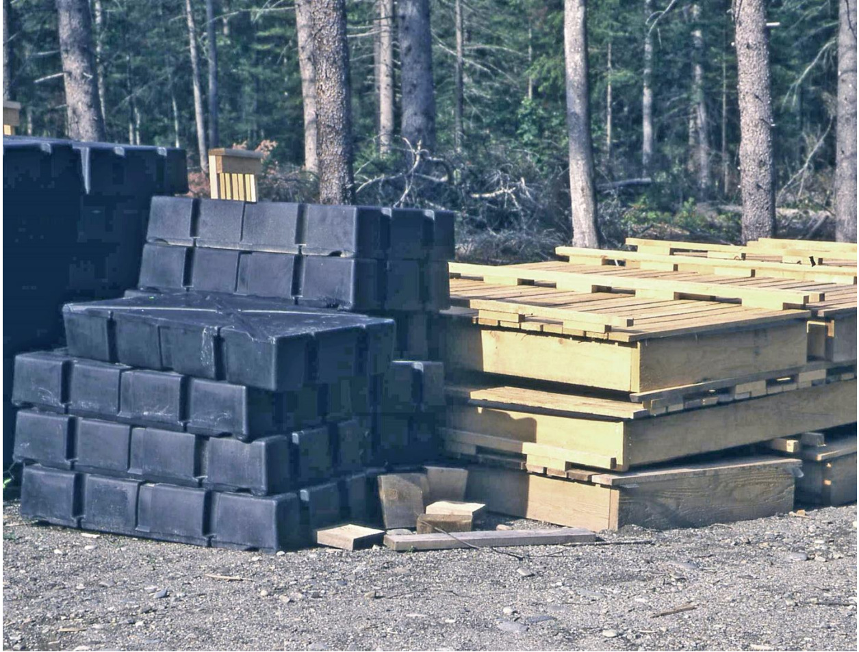
Fig. 18. Floats and sections stockpiled at assembly site. Floats are 4 x 2 x 0.67 ft (~1.2 x 0.6 x 0.2 m). Ronald B. Davis photo.
